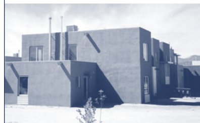
The Ohkay Owingeh Housing Authority used USDA Rural Development Section 515 funding to develop rental homes on the San Juan Pueblo in northern New Mexico.
