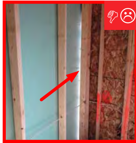
B./C. Common wall sheathing not properly fastened or sealed.
