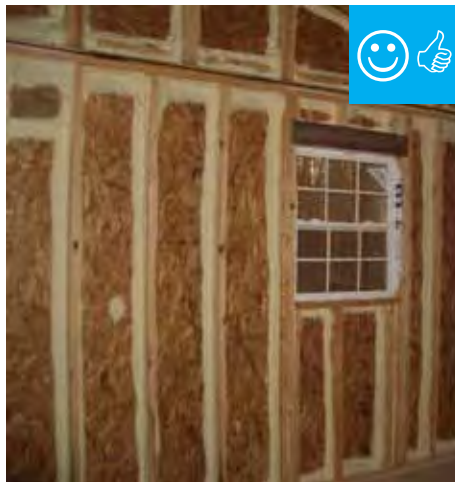
Air barrier is air sealed.
