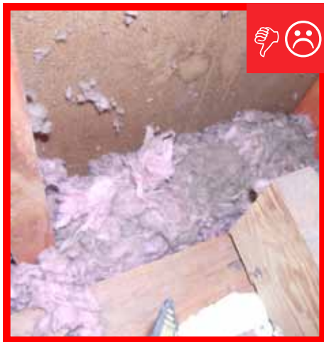
B. Wall from above without top plate or blocking installed.
