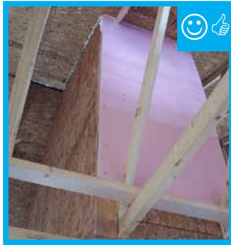
Rigid air barrier is installed to hold insulation in place.
