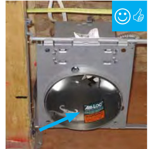
ICAT labeled recessed light installed but still needs gasket.
