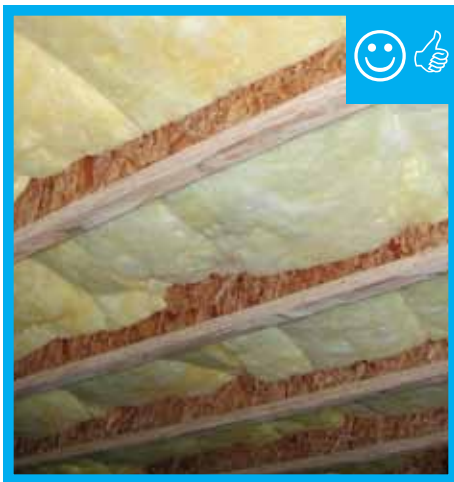
Insulation is in contact with floor above.
