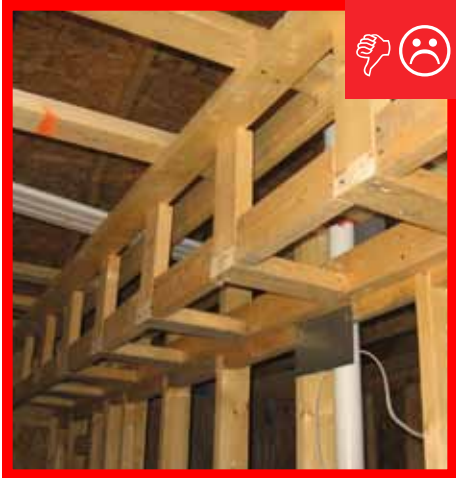
A. No air barrier is present between the dropped ceiling/soffit and the attic.
