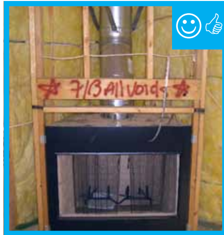
Insulation installed behind fireplace prior to air barrier installation.
