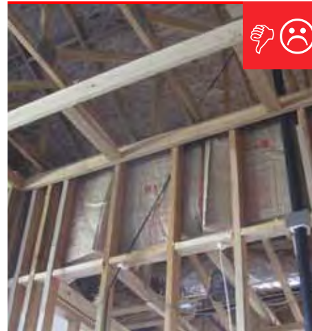
B. No rigid backing on knee wall.
