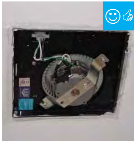
Fan with a cleanly cut and properly sized hole has been air sealed to drywall.
