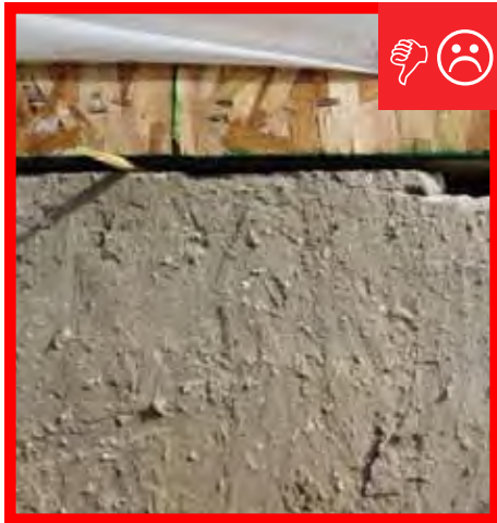
A. No foam gasket or air seal between sill plate and masonry foundation.
