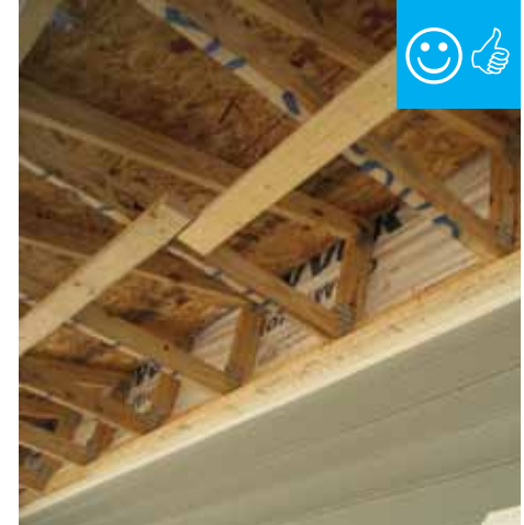
Air barrier is installed prior to porch attic framing.
