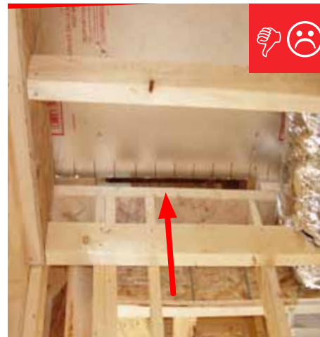
B. Seams of air barrier not sealed.
