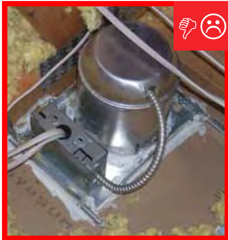
A. Non ICAT recessed light installed.
