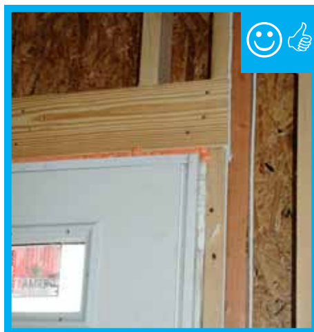
Appropriate door framing installed.
