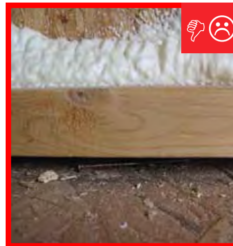
B. Foam sprayed at exterior sheathing and sill plate connection leaving gaps beneath sill plate.
