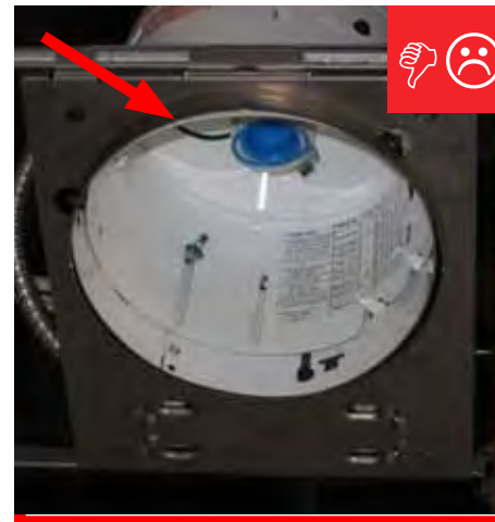
C. No gasket installed.
