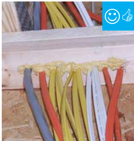
Wiring penetrations have been neatly sealed with foam.
