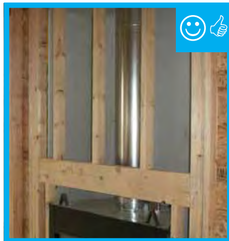
Rigid air barrier is installed behind fireplace.
