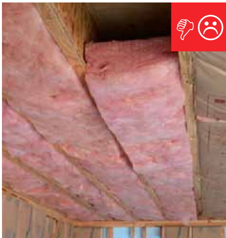
C. Insulation is misaligned with floor above.
