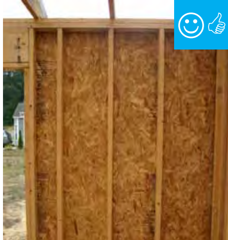
Proper spacing of 2 x 4 studs.
