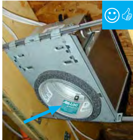
ICAT labeled recessed light with trim kit installed.
