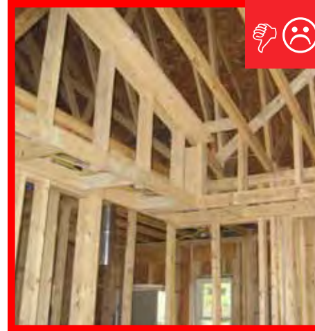
A. No air barrier is present between the dropped ceiling/soffit and the attic.
