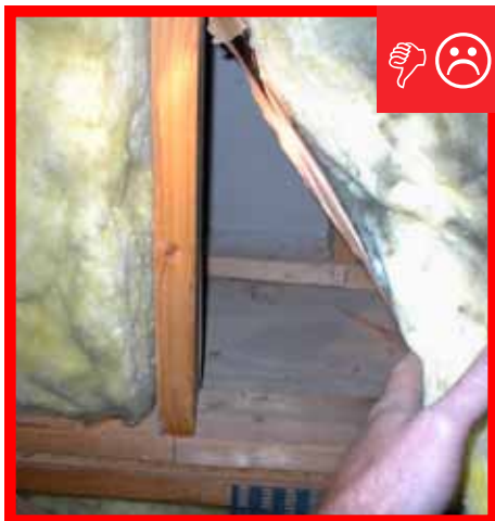
C. Insulation does not fill entire cavity nor is there an air barrier present between the double wall.
