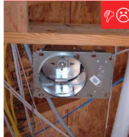
A. Non ICAT recessed light installed.
