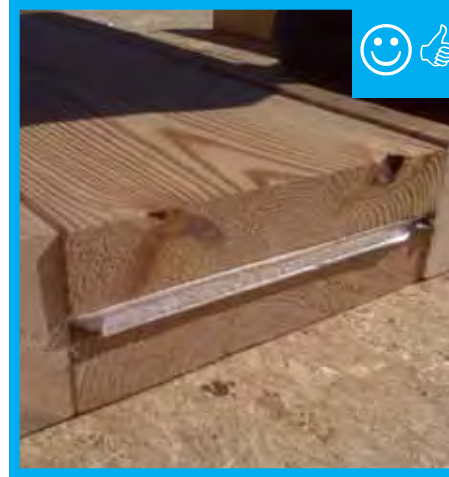
C. Verify two member headers with rigid insulation between are installed.
