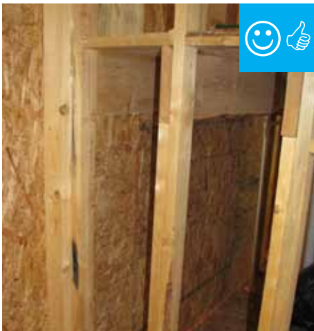
Air barrier installed under staircase.
