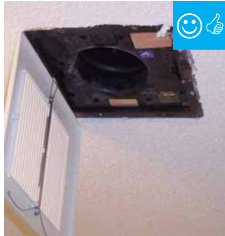
Cleanly cut and properly sized hole.
