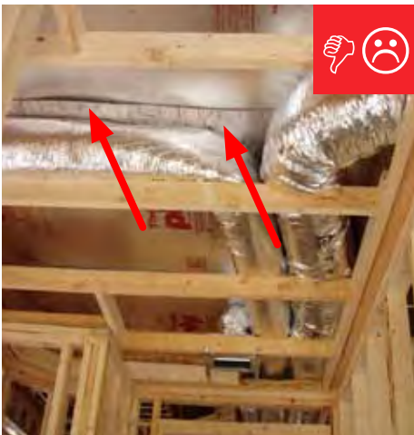
B. Seams of air barrier not sealed.
