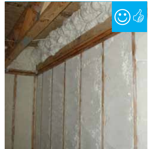
RESNET Grade I installation of spray foam insulation.
