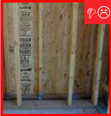
A. No air barrier installed between the walls and a larger gap between the walls that needs sealing.
