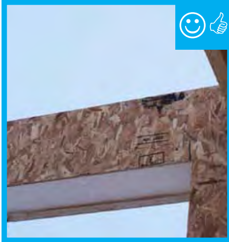
B. Verify SIP headers are installed.
