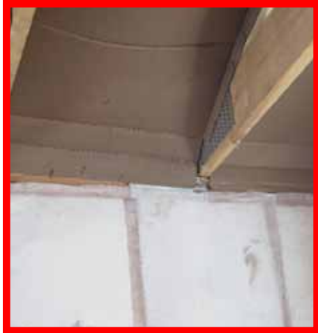
A. Wind baffle installation will not allow insulation over the top plate.
