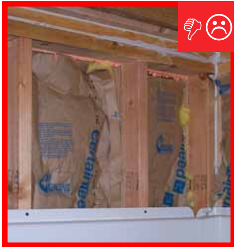
A. No air barrier installed between double-wall framing.
