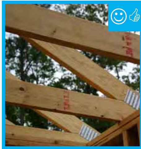
Framing allows for required insulation depth.
