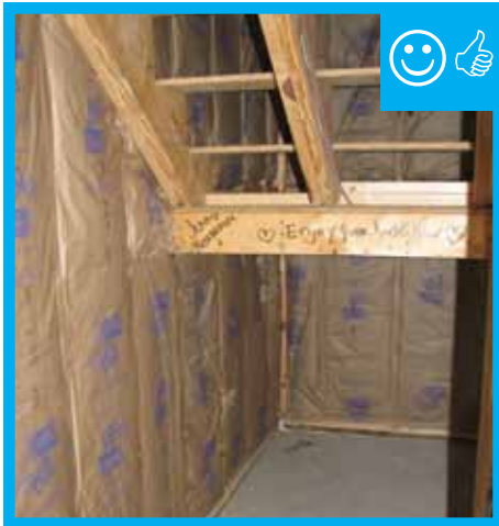
A. Insulation properly installed before air barrier.
