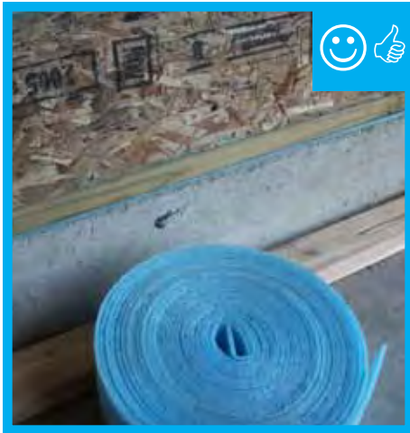
Foam gasket installed between sill plate and foundation.
