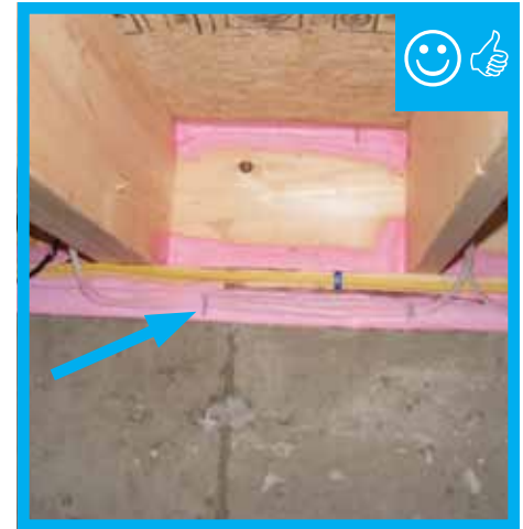
Sill plate was sprayed with foam prior to installation atop foundation.
