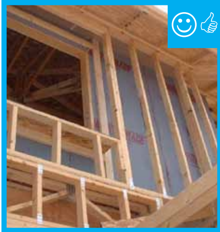
Rigid air barrier installed between double-wall assembly. Inside cavity will be insulated.
