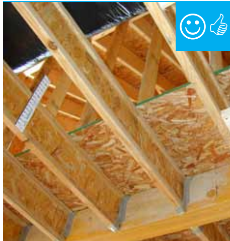
A. HVAC platform installed to allow for proper insulation depth.
