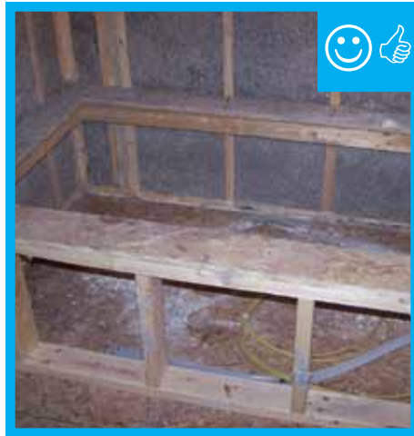
Insulation meets RESNET Grade I prior to air barrier installation.
