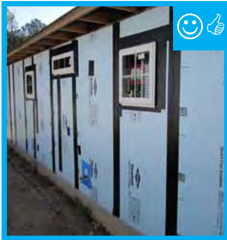
A. Continuous rigid insulation has been installed.
