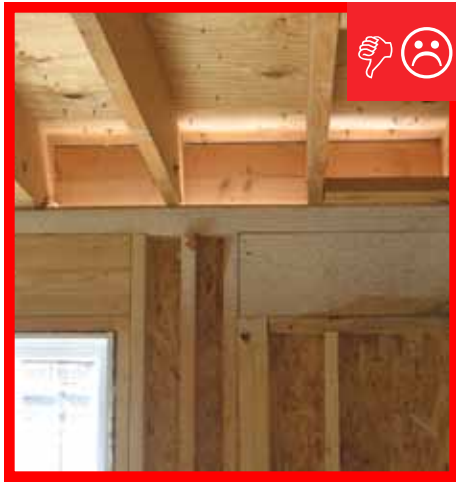
A. No air barrier is present between cantilever and conditioned space.
