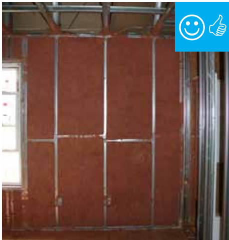
RESNET Grade I installation of blown insulation.
