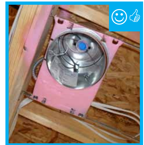
ICAT recessed light sprayed with foam to act as gasket against the drywall.
