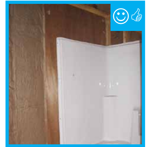
Air barrier installed behind shower stall.
