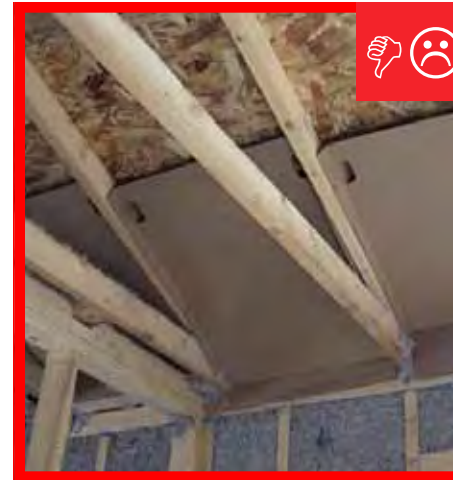
A. Framing and wind baffle installation will not allow for required insulation depth.
