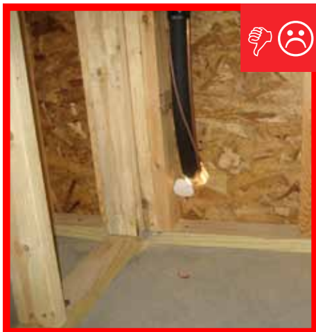
B. Hole has not been air sealed.
