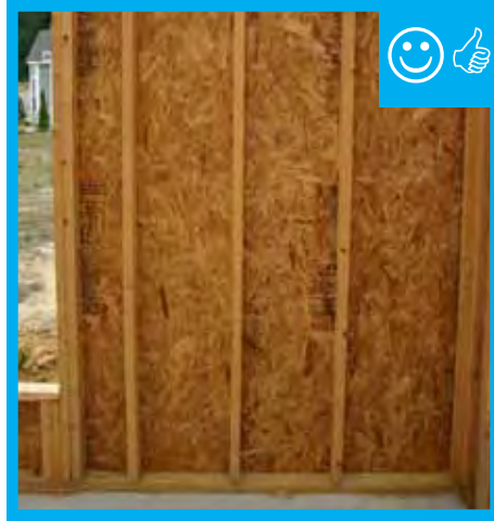
Continuous air barrier
