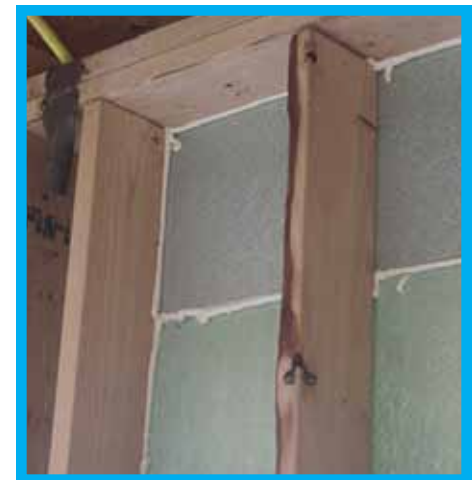
D. Insulated sheathing has been taped and sealed at seams.
