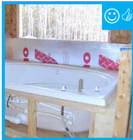
Air barrier installed behind the tub.
