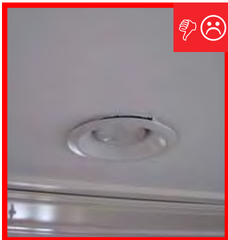
B. Recessed can light has not been sealed to drywall.
