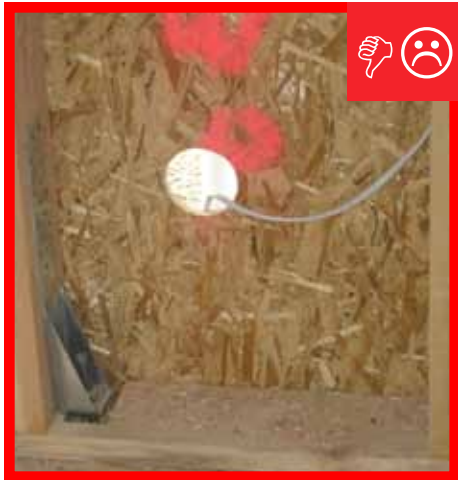
A. Holes have been cut excessively larger than needed making it difficult to seal.
