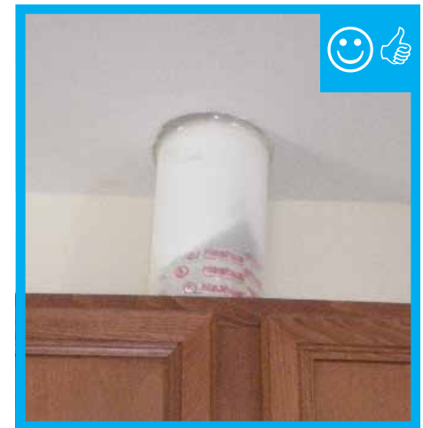
Kitchen exhaust penetration has been sealed with caulk.
