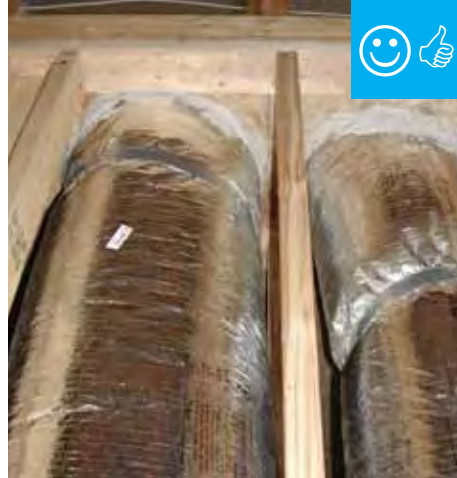
Chase capped with rigid air barrier and duct work penetrations properly sealed.
