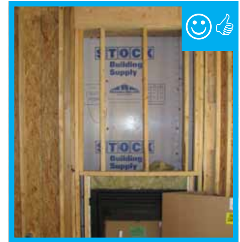
Rigid air barrier is installed behind fireplace.
