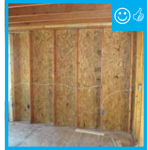
Proper spacing of 2 x 6 studs.
