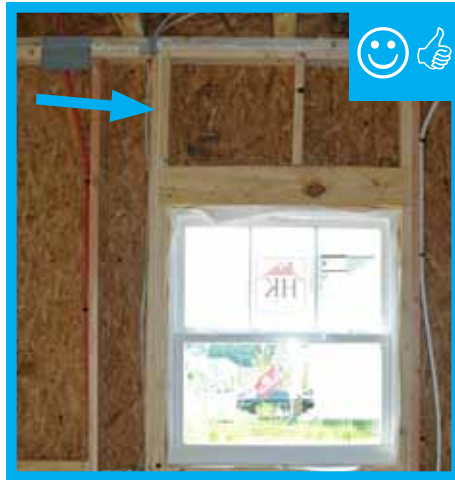
Window framing has appropriate number of king studs.
