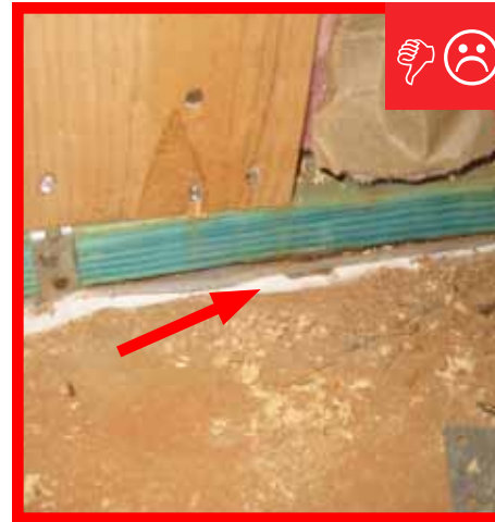
A. Caulk is too far from sill plate to properly air seal.
