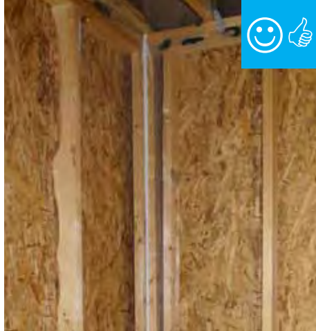
Framing allows for corner to be insulated.
