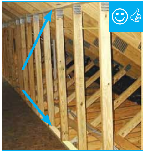
Top and bottom plates installed prior to backing and insulation.
