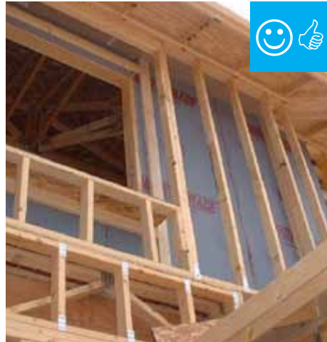
Air barrier is installed between double-wall framing.
