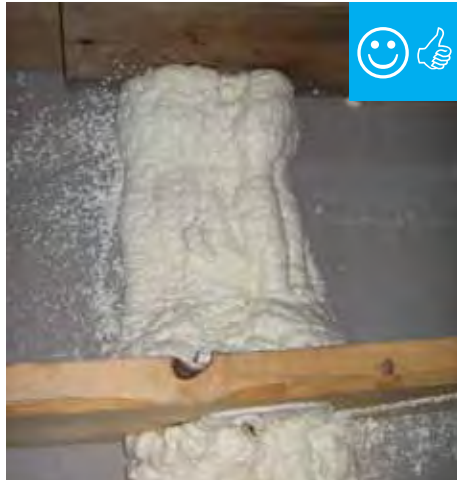
Top plate to drywall connection sealed from attic with foam.
