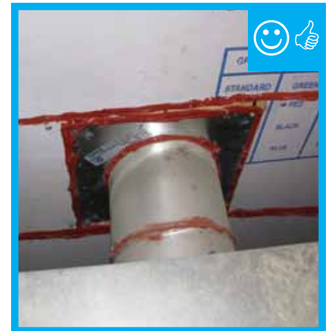
Vent and air barrier sealed.
