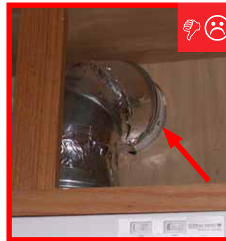
B. Kitchen exhaust has not been air sealed.
