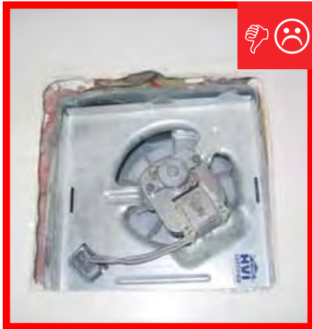
A. Roughly cut hole that is larger than the fan making it difficult to seal.
