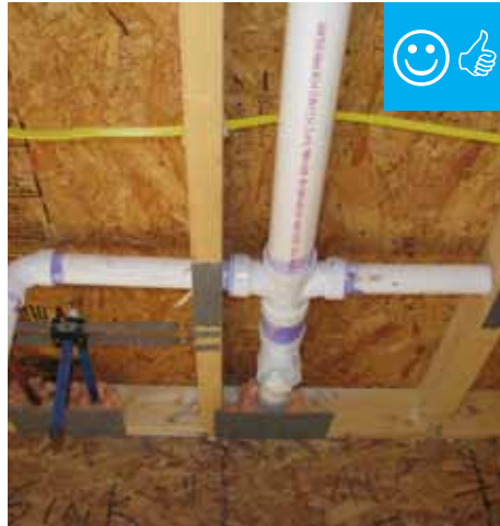
Neatly cut hole has been properly sealed with foam.
