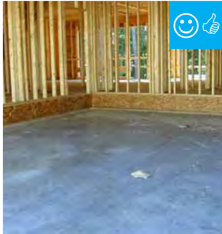
Air barrier is present between garage and floor system.
