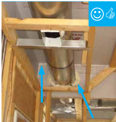
Seams and penetrations of air barrier properly sealed
