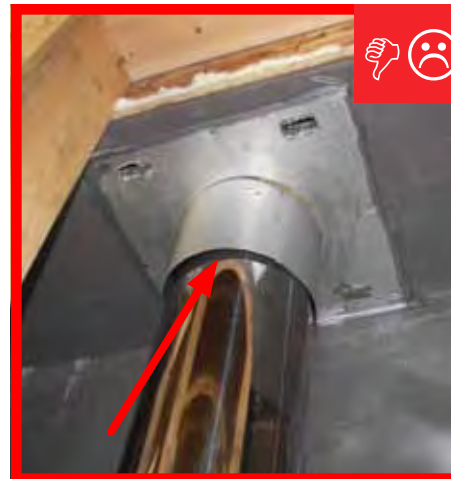
D. Vent sleeve not completely sealed.
