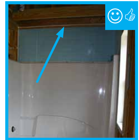
Air barrier sealed.
