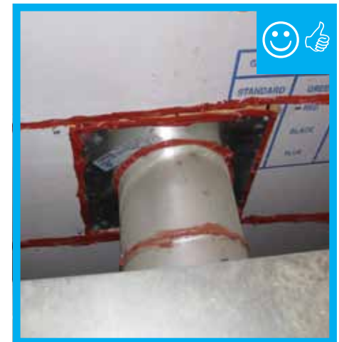
Vent and air barrier sealed.
