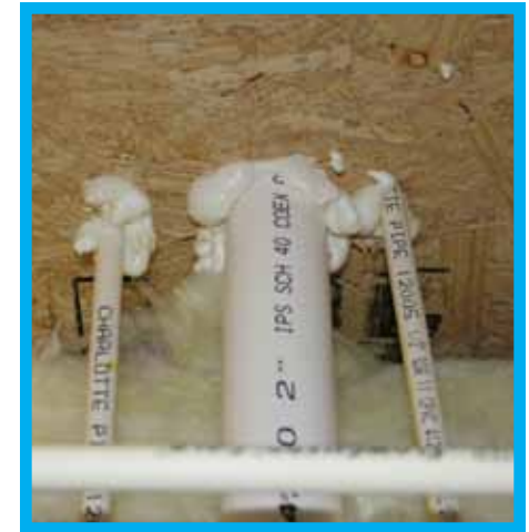
Penetrations through floor are air sealed.
