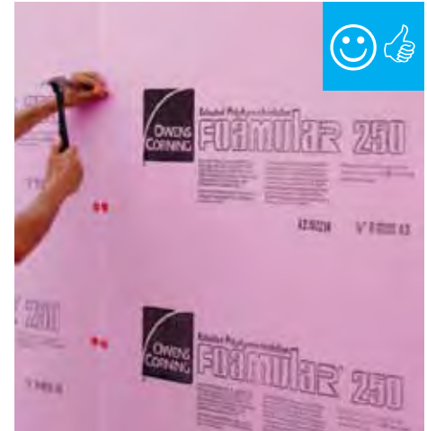
Rigid insulation is being installed with cap nails.
