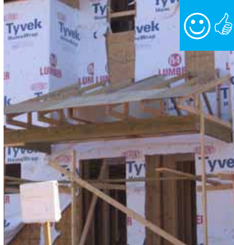
Air barrier is installed prior to porch attic framing.
