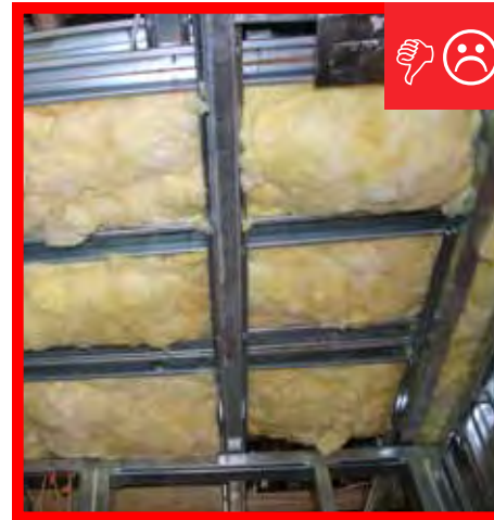
B./C. Insulation will not be aligned with air barrier.
