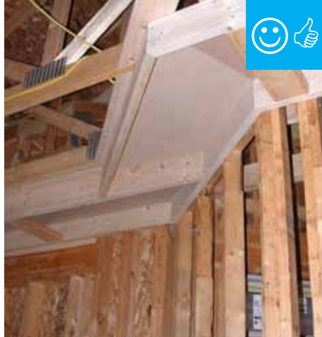
Air barrier is present between the dropped ceiling/soffit and the attic.
