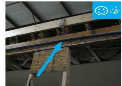
Gasket installed at marriage wall connection prior to assembling modules.
