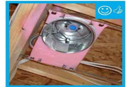
ICAT recessed light sprayed with foam to act as gasket against the drywall.
