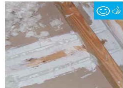
Top plate to drywall connection sealed from attic with caulk.
