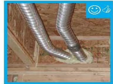
Neatly cut and sealed penetration.
