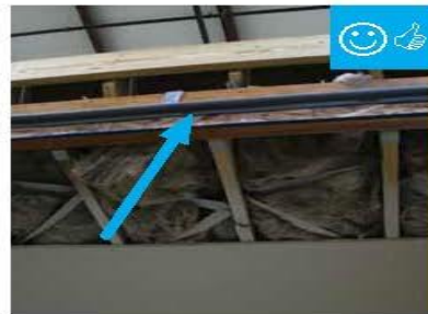
Gasket installed at marriage wall connection prior to assembling modules.
