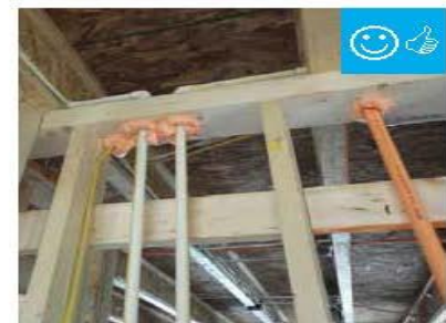
Neatly cut hole has been properly sealed with foam.
