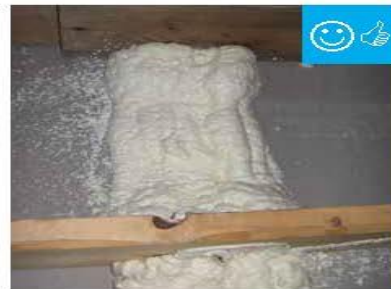
Top plate to drywall connection sealed from attic with foam.
