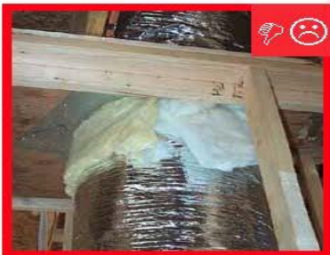
C. Fibrous insulation does not air seal.
