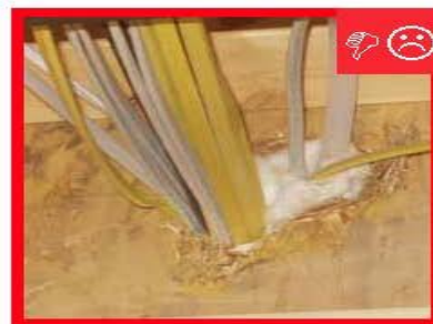
B. Fibrous insulation is not an air barrier and cannot be used for sealing holes.
