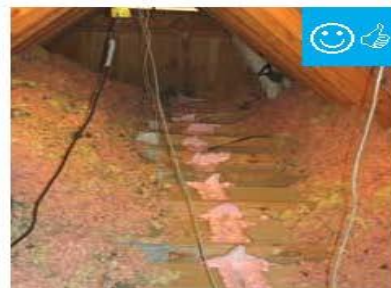
Top plate to drywall connection sealed from attic with foam sealant.
