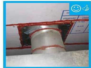
Vent and air barrier sealed.
