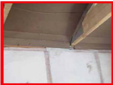
A. Wind baffle installation will not allow insulation over the top plate.
