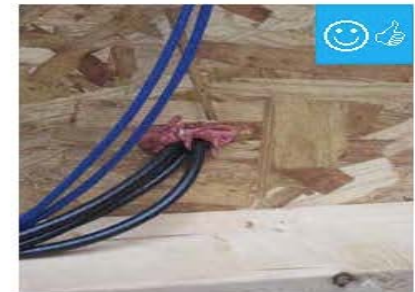
Wiring penetrations properly air sealed.
