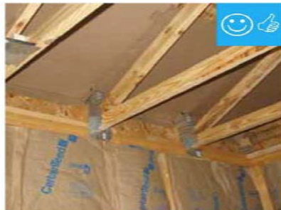
Wind baffle installation will allow proper insulation depth over the top plate.
