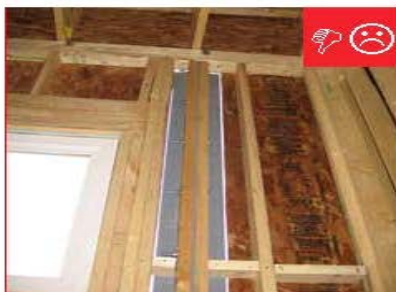
B. Air barrier is air sealed.
