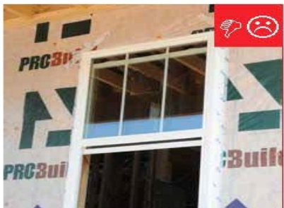
A. Window does not meet 2009 IECC requirements.
