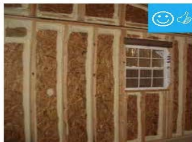
Air barrier is air sealed.
