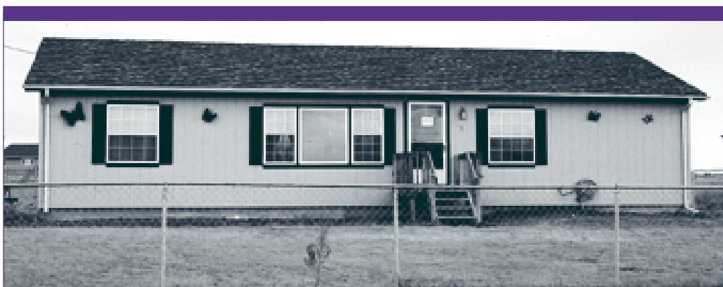
This new home in Pine Ridge Village was constructed through OSTPH's self-help program.
