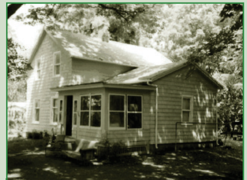
Sheen Housing renovated this home to improve its indoor air quality and efficiency.
