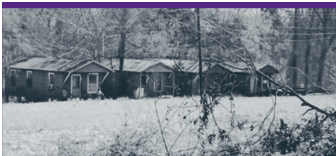
“Shotgun houses” are prevalent in the Mississippi Delta, including West Feliciana Parish.
