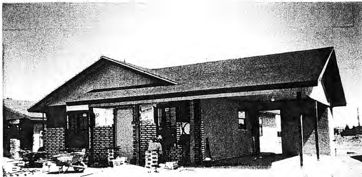
Figure 2c: Construction of Tierra Linda Phase I
