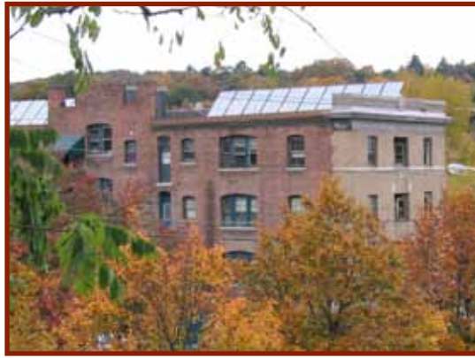
At the Abbott Block in Brattleboro, Vermont, solar panels are expected to save 50 percent annually on domestic hot water. The panels preheat the water supply for 17 apartments, including 2 units in an adjacent building. Other improvements included new energy-efficient windows with low-E glass, 9 inches of hard insulation added to the roof, new ENERGY STAR® appliances, low-flow plumbing fixtures and laundry equipment, and new lighting fixtures and bulbs. Overall, energy retrofit work is expected to save 25–30 percent in operating costs. Photo provided by Windham Housing Trust.
