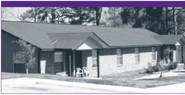
Feliciana Hills Apartments provide one-, two- and three-bedroom units to low- and moderate-income families in the parish.
