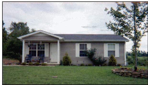
Figure 1. The young homeowner's new home, built by KMHDC.
