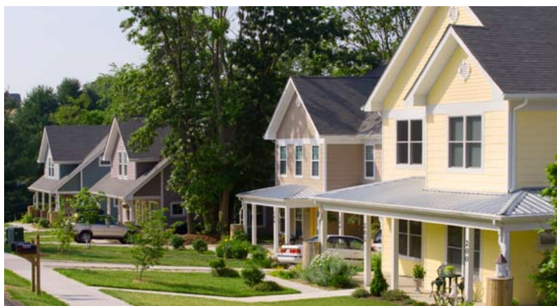
The fourteen ENERGY STAR® qualified units of the Roanoke-Lee Street project received an average score of 75 on the HERS Index.
