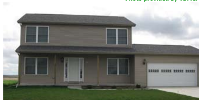
This ENERGY STAR® home built by YBMC's self-help program earned a 75 on the HERS Index.
